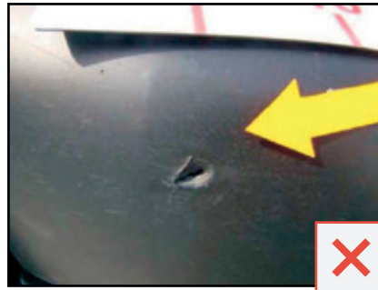
Excessive, apparent damages on the non-painted bumpers are not acceptable.
